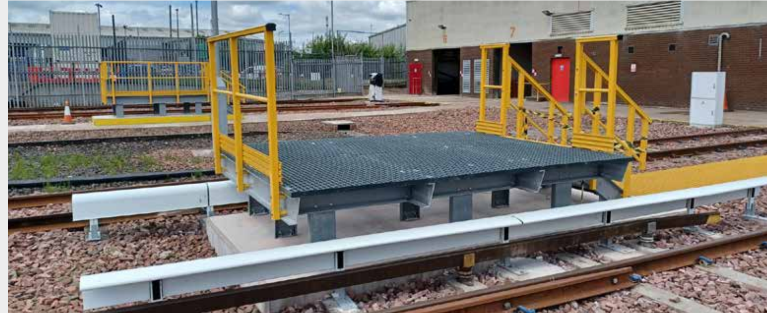
Installation of access / egress platforms for use with the new trains.
