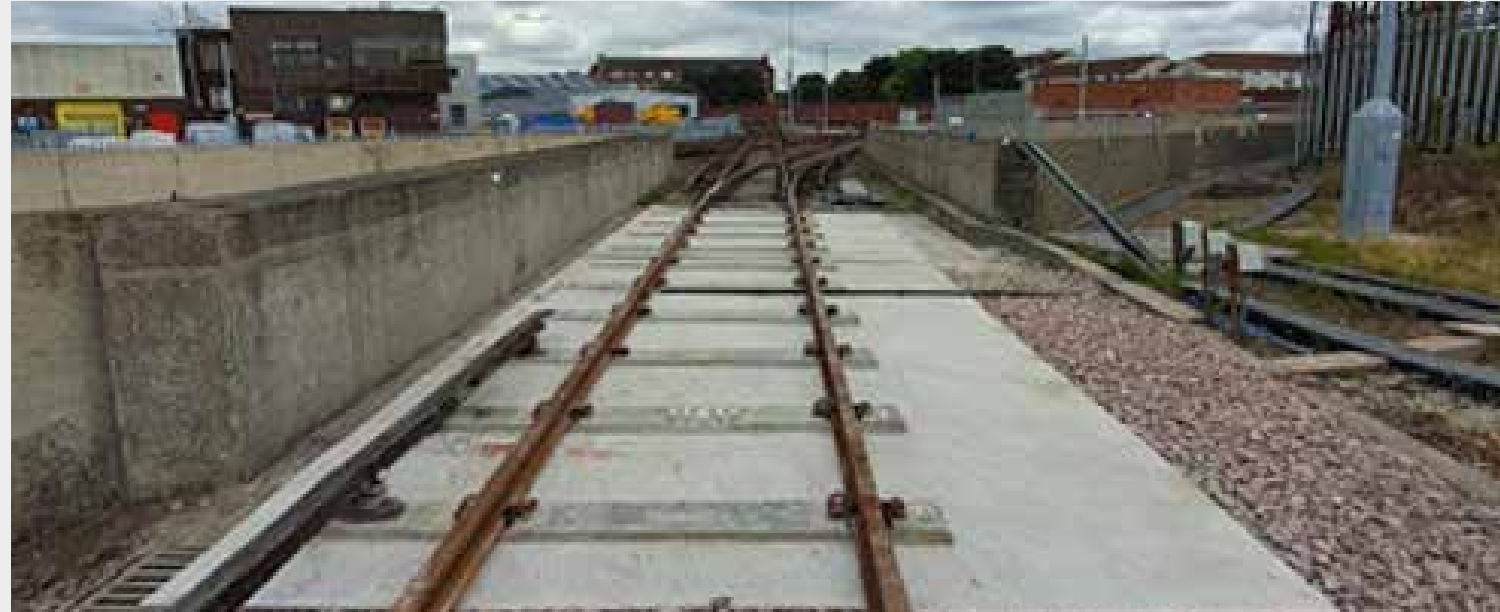
Overbridge track renewal.
