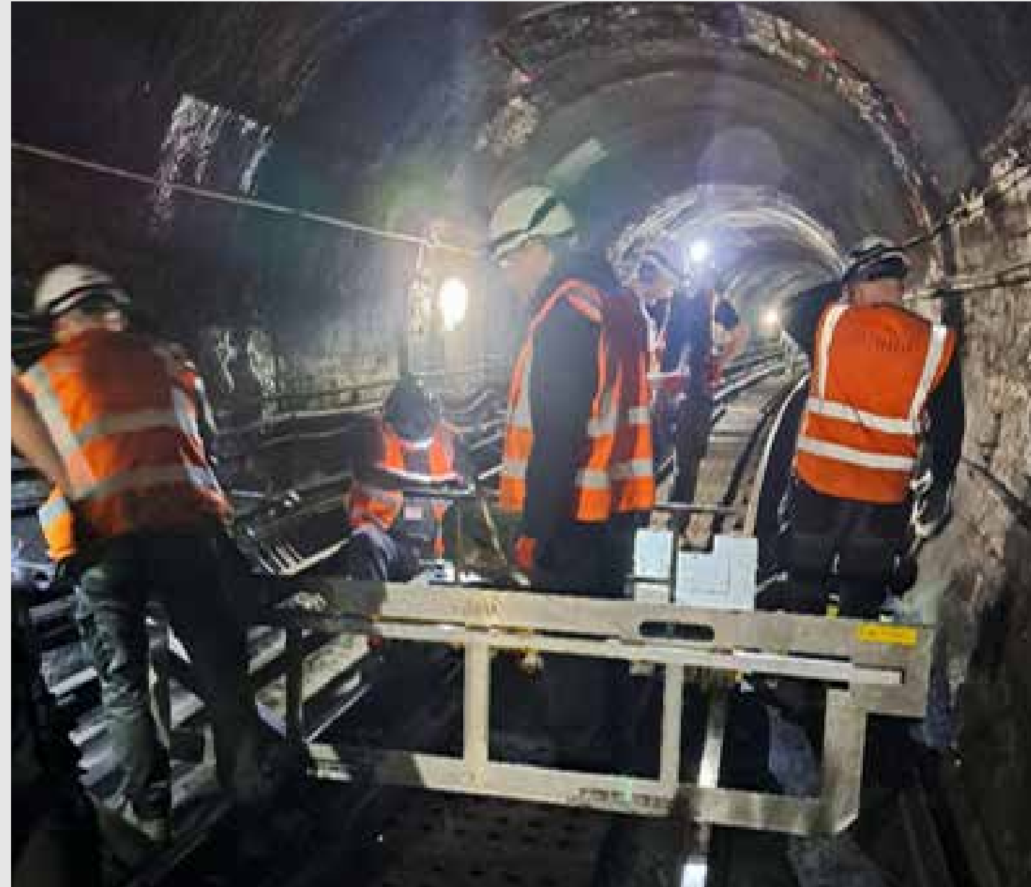
Waveguide and tunnel cabling installation progress good.
