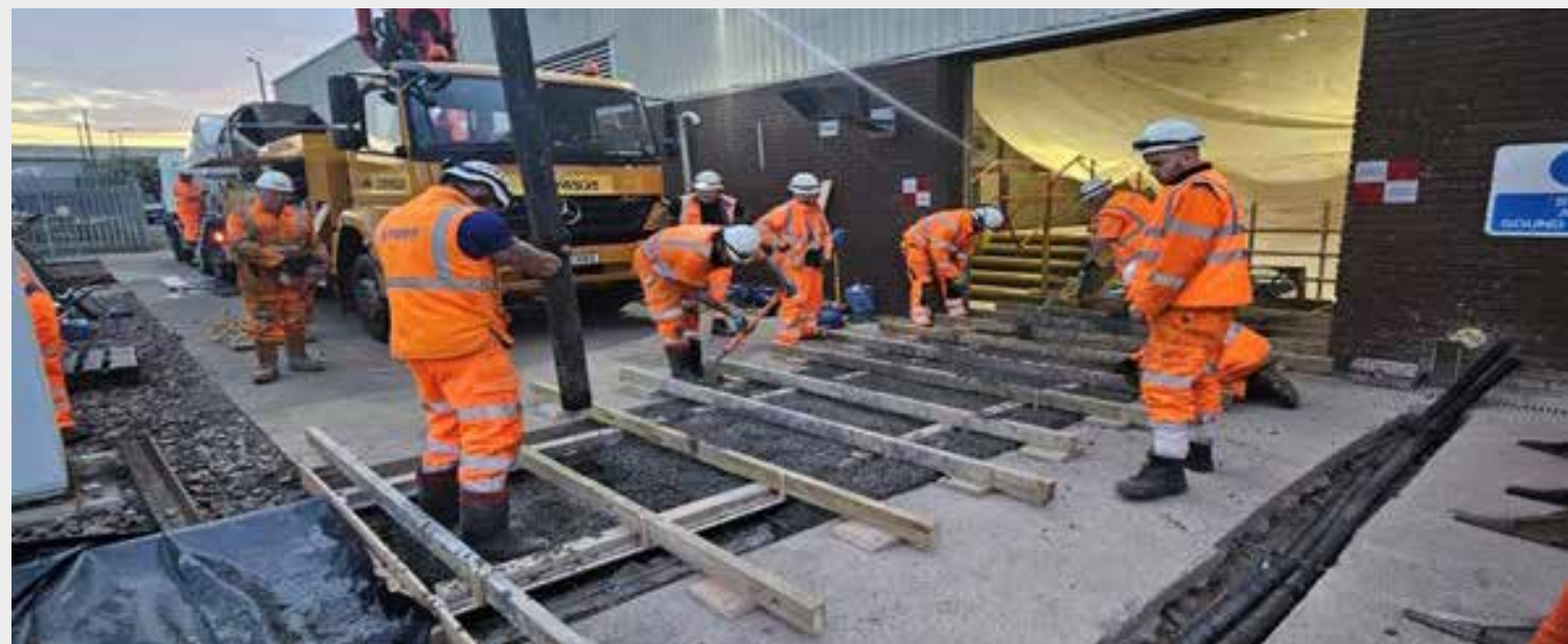
Maintenance Shed works to improve track alignment & replace embedded rail.
