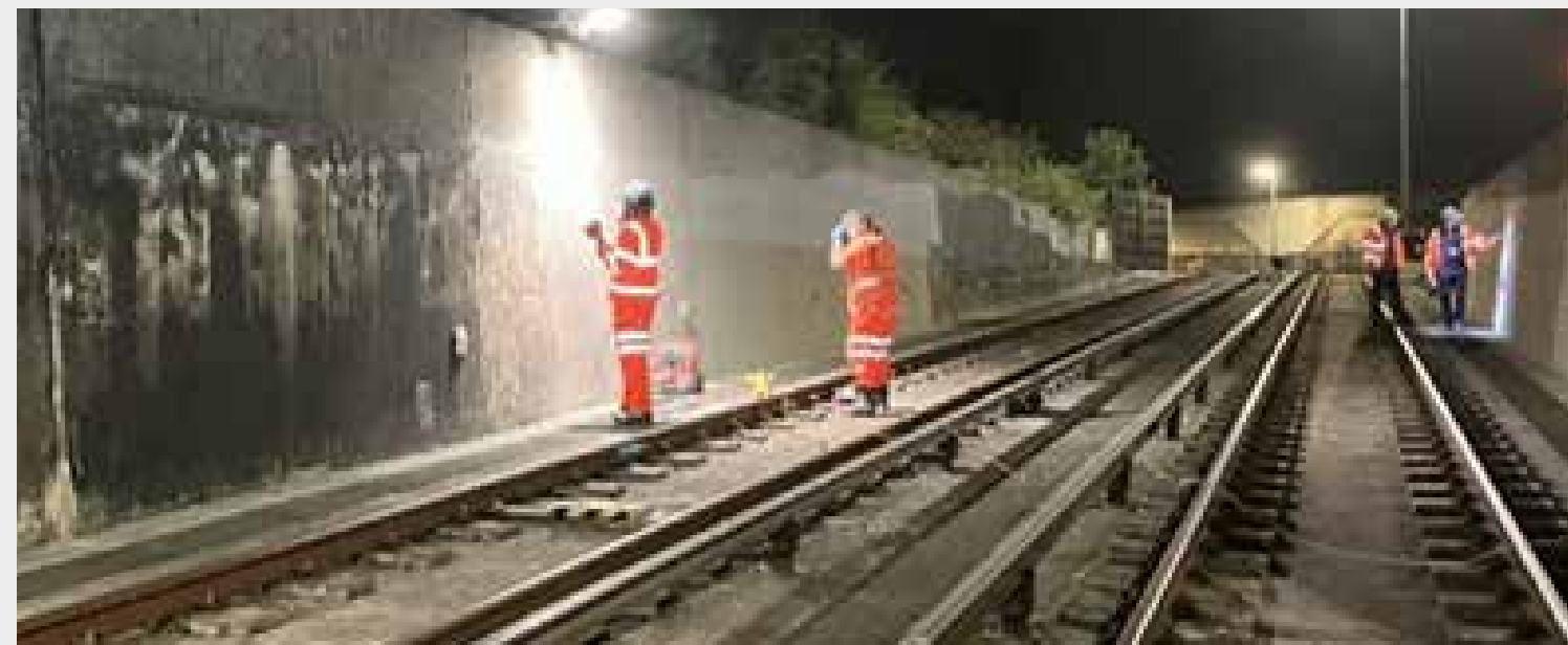
Ramp retaining wall concrete repairs.
